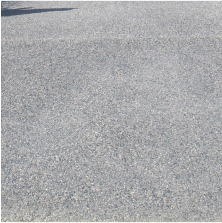
Primary Path - Exposed aggregate concrete
